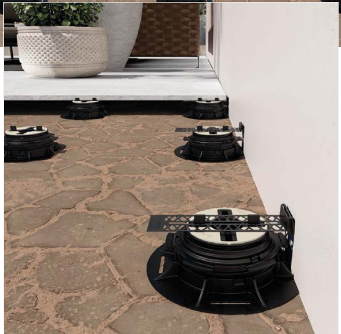
A Perimeter Spacer is placed on top of the self levelling head and two pre-cut flaps removed on pedestals at the edge of the tiled area.
